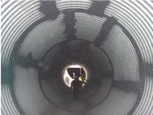
Watercourse and drain culverts
